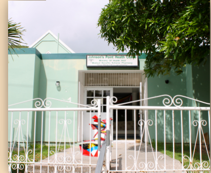
Johnson's Point Health Centre
